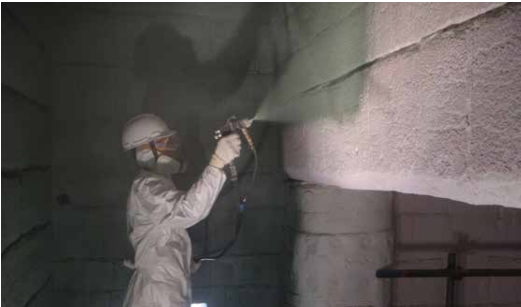
emisspro® – an industrial furnace refractory coating
